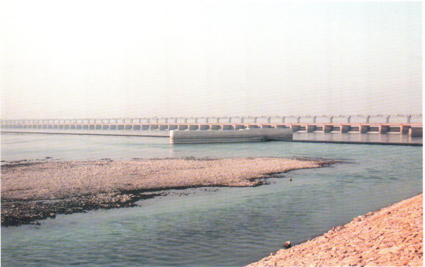
Fig. 1. Downstream of Jinnah Barrage.
